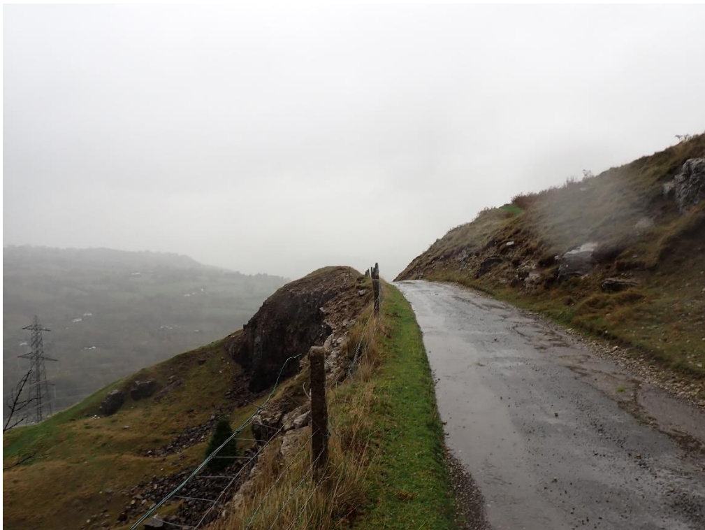
Plate 22: Chainage 199m, crest of slope / rock face close to edge of road. Note the poor quality of the fence.
