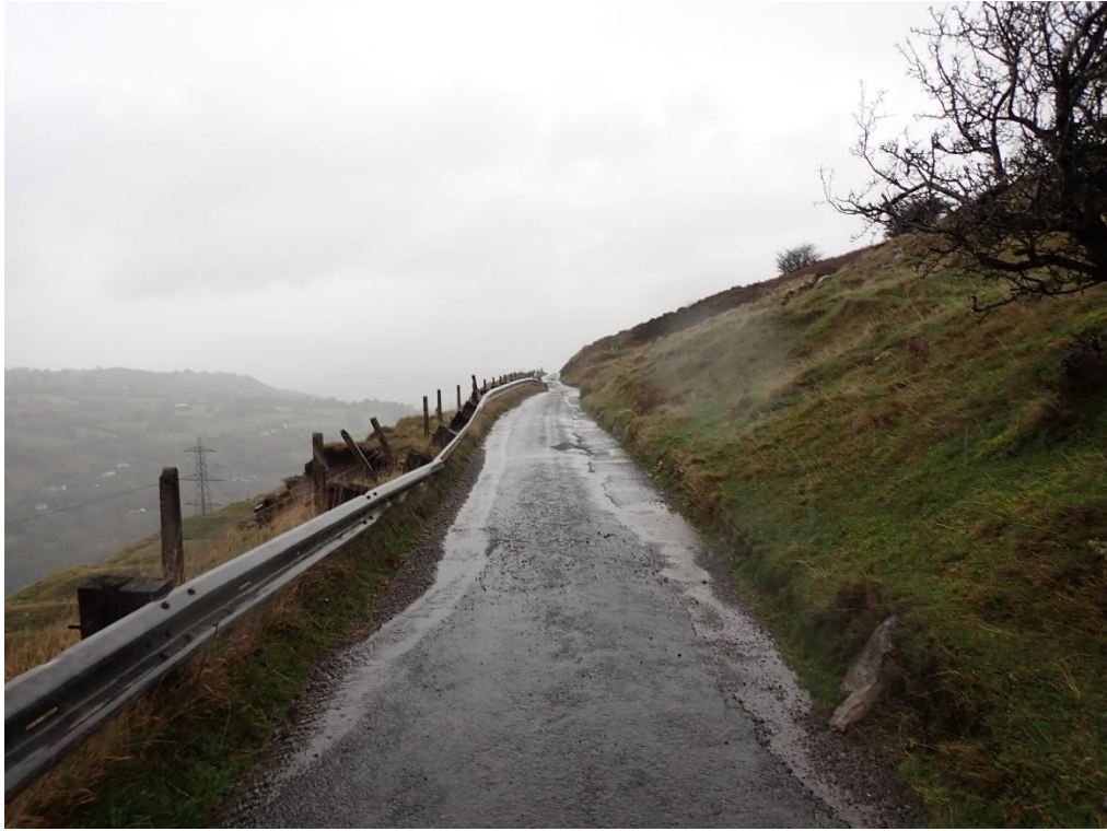
Plate 11: Chainage 90m, VRS section starts.
