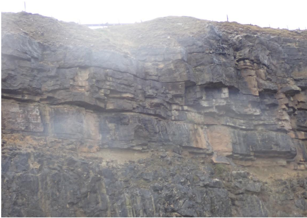
Plate 30: upper rock section with rockfall debris on ledge of weaker materials (recent rockfall).
